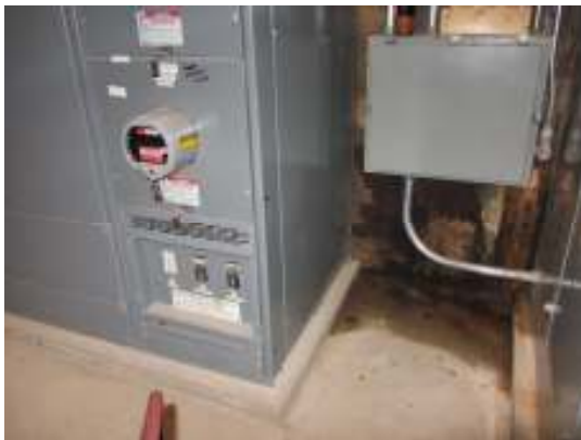
Active water leak at basement foundation wall in electrical room
