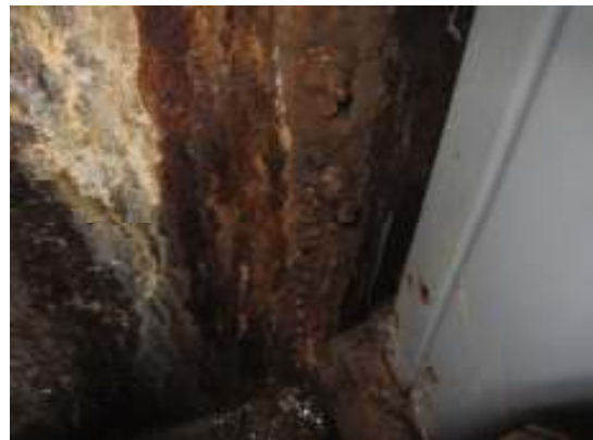
Active water leak at basement foundation wall in electrical room
