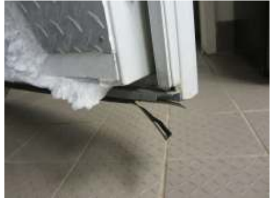
Main freezer walk-in door seal damage resulting in interior frosting
