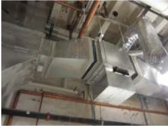
Air gaps noted at basement air plenum ductwork
