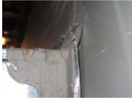
Air gaps noted at basement air plenum ductwork
