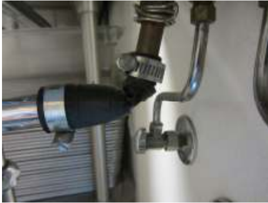
Basement sink drain vent line kinked
