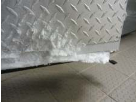
Main freezer walk-in door seal damage resulting in interior frosting
